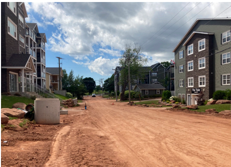
Harley Street Rehabilitation Upgrades to Harley Street included new stormwater measures and water/sewer pipes as well as new sidewalks and chicanes to assist in traffic management.
